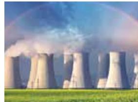
Nuclear Power Plant
